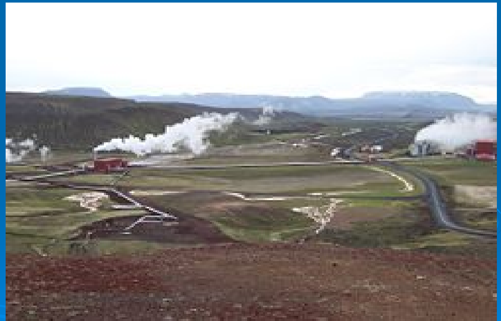
Krafla Geothermal Station in northeast Iceland
