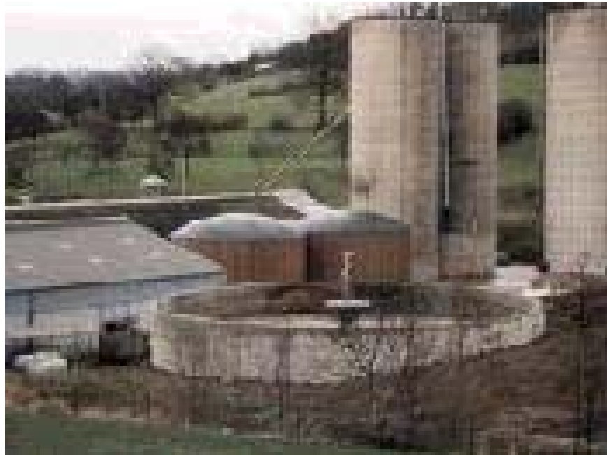
Photo 2.2: Biogas plant at Mauternach – Luxembourg (Gas production: 1000 m 3 /d, Generator: 1x50 kW, 1x 75 kW)
