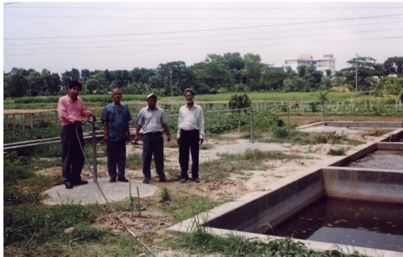
Photo 3.4: Poultry-based biogas plant at Faridpur Muslim Mission being visited by the Study Team
