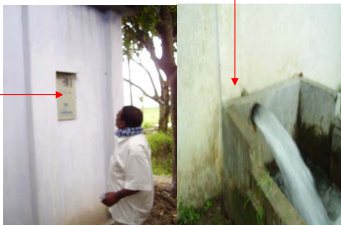
Photo shows Flow of Irrigation Water to the Field after SMART CARD inserted by the Farmer /Pump.
