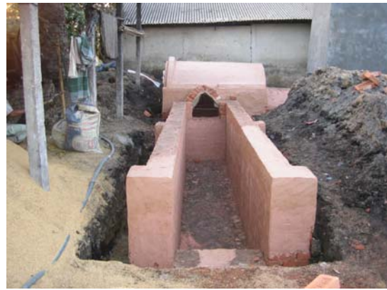
(b) Chimney under construction at Kaliakoir
