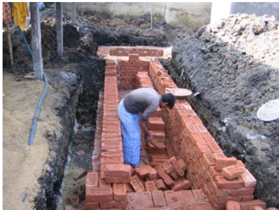
(a) Chimney base construction at Kaliakoir
