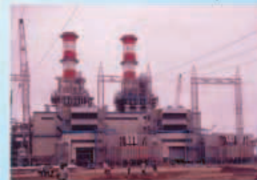
450 MW Meghnaghat Power Station, financed by IDCOL.
