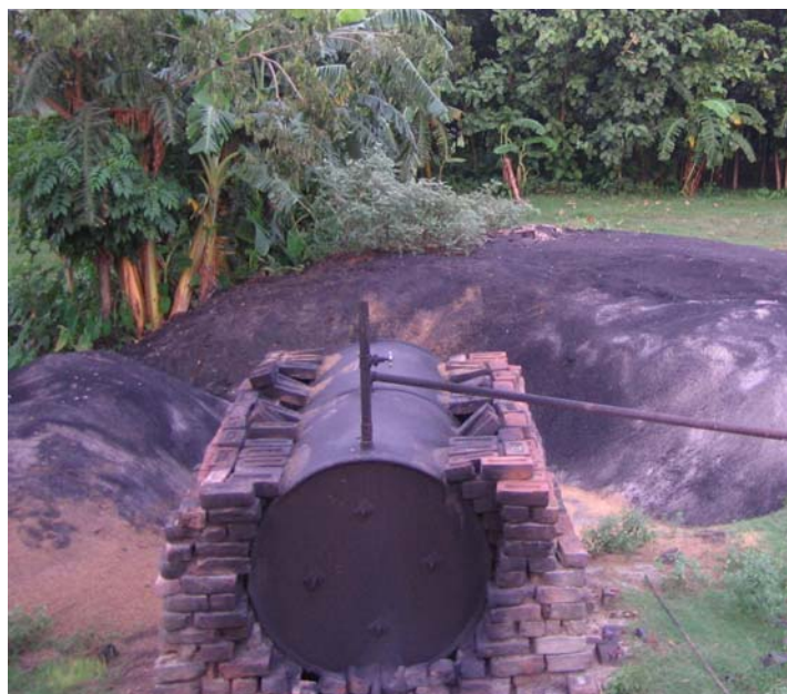
Photo 3. Local made cylindrical steam generator
