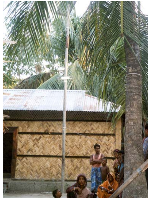
Figure 3: PV module installed on the bamboo with no concrete support
