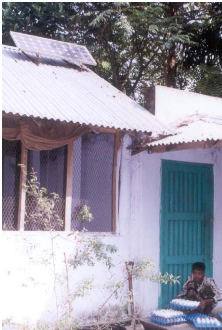
Figure 2: PV module installed on the roof with simple mounting support
