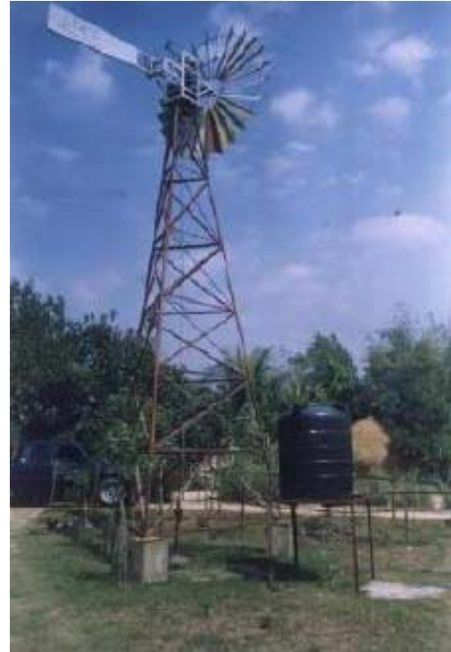
Typical Water pumping Windmill, Sherpur District
