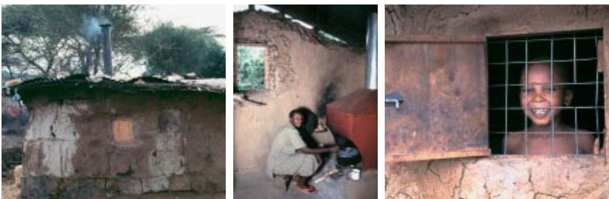
Interventions to the living environment being developed in rural Kenya: (Left): enlargement of windows in traditional Maasai home. (Middle): hood with flue, enlarged eaves spaces and enlarged and better positioned windows. (Right): smoke vented from the home through a hood with flue. See Case Study 3 (next page) for further explanation.
