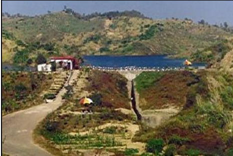
10 kw Micro Hydro Power Unit, Bamerchara, Banshkali, Chittagong
